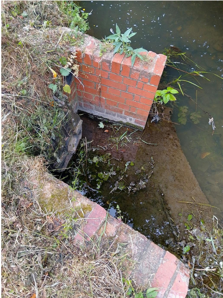
Photo 18. One of two adjacent storm overflow drains (51.903289 , -2.0874793). What gets discharged to the watercourse from these drains is always a big concern. Obtaining a services map of pipework to review the likely inputs will help understand water quality impacts to the Chelt. GORC can also actively monitor upstream and downstream during periods the pipe is running. Concerns would be contents of road run off (microplastics and pollutants) and misconnections in residential properties (washing machine phosphate input). Mapping features like this and engaging the Council may provide opportunity to break these out (space provided) and run through an urban sustainable drainage system feature (SUDs – e.g. swales, retention pools etc) to allow the water to settle out fine sediment and contaminants a little before reaching the river. Examples such as the 'Outfall Safari' highlight where community groups have mapped issues before: https://www.southeastriverstrust.org/projects/outfall-safaris
