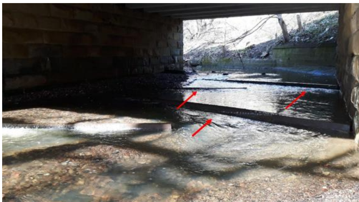
Figure 5 Alternatively, a series of low baffles can be installed in a culvert to create depth and flow conditions allowing fish to pass through at low flows (red arrows highlight the baffles)
