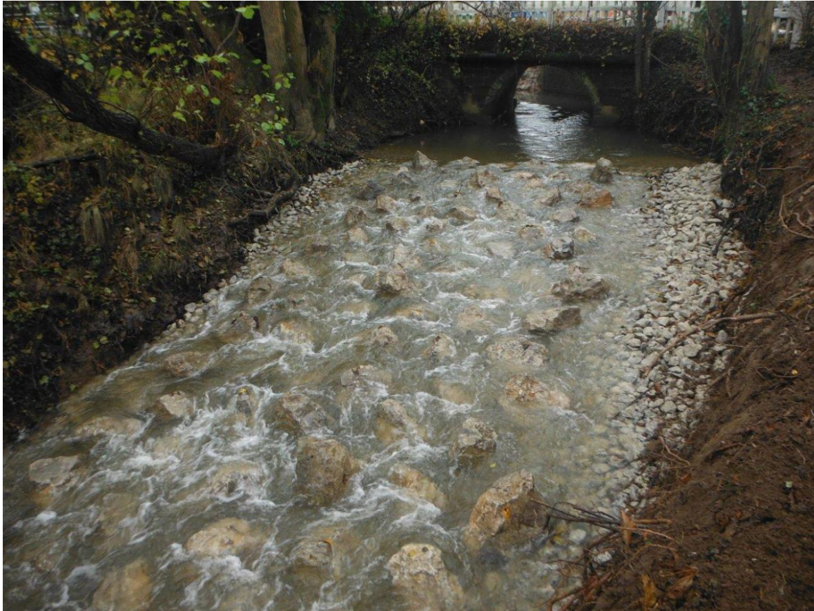
Figure 7 Example of a rock ramp. It could be possible for the concrete in the overflow channel between Honeybourne Way and the weir to be chopped out, reformed and a rock ramp installed across the gradient between the Chelt downstream on the road culvert – buried underground service cables and pipes allowing. Alternatively, a technical fish pass could be investigated, but these are very expensive to install and need maintenance. Baffles at the entrance to the culvert may be required to maintain water depths and velocities to enable fish passage. It may be a variation on this solution could be used at the top of the overflow channel to get fish up to the Waitrose car park culvert.
