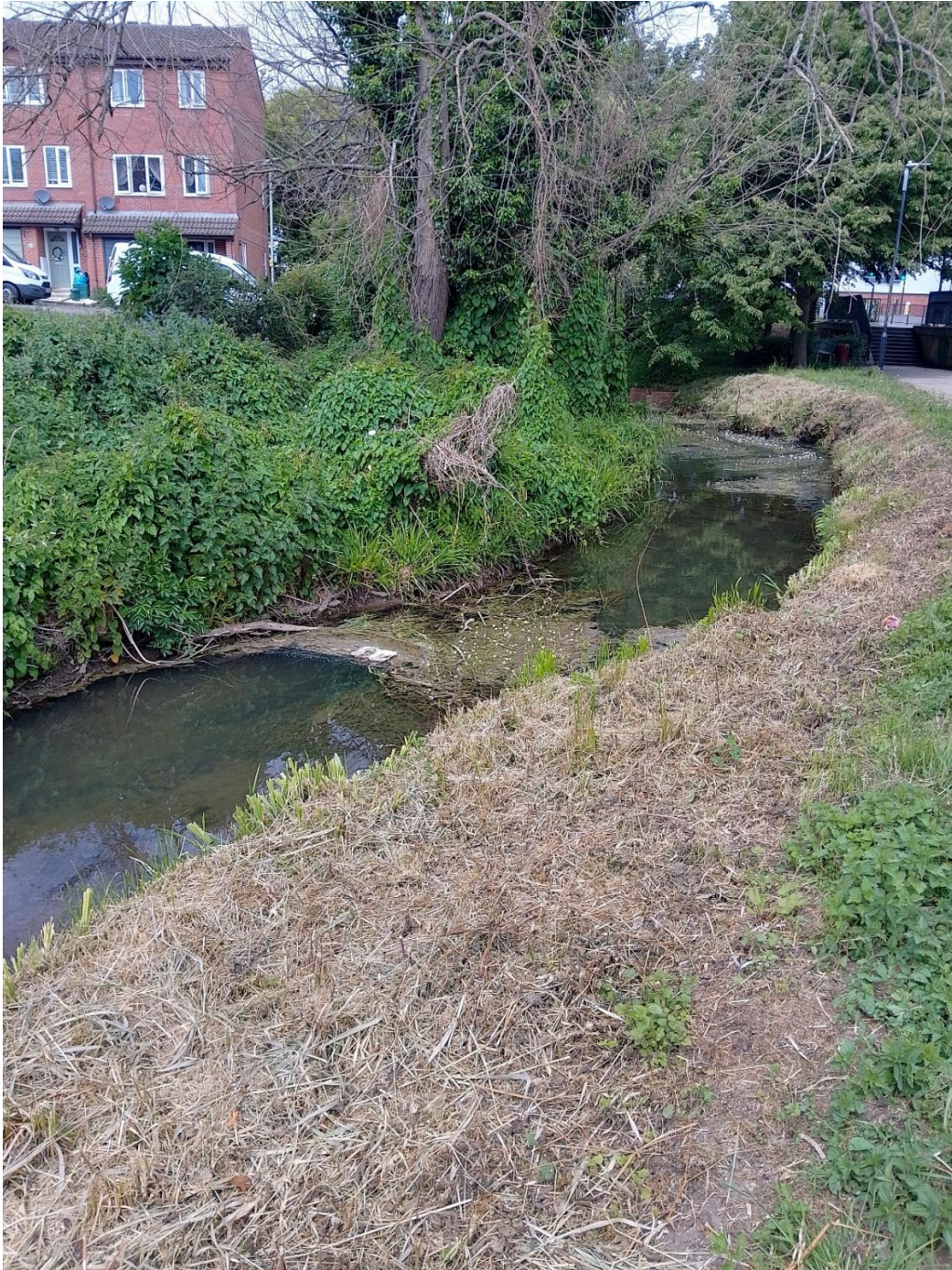
Photo 22 The end of the section of Chelt reviewed at Gloucester Road. The end of the channel that can be seen in the middle distance becomes quite constrained and a small brick wall interacts with the channel. This should be reviewed to avoid any influence on flood water being backed up by the constraint here.
