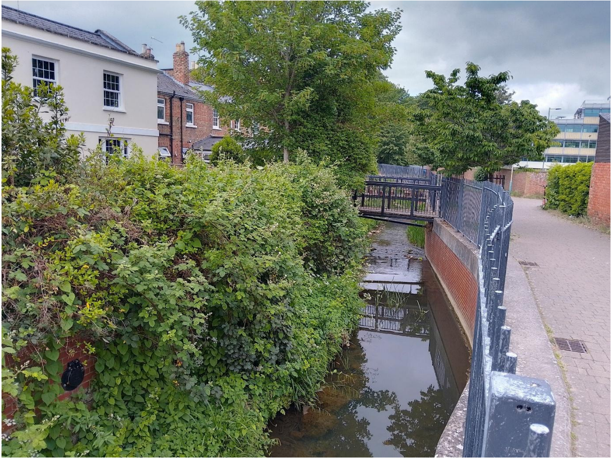
Photo 2 The deeply incised channel also has its movement limited by the high brick-built walkway on the RHB. Water velocities through this section are likely to be difficult as levels rise and flows speed up; the smooth brick wall provides little resistance to slow the water down. The summer vegetation on the LHB will provide some flood water refuge to aquatic wildlife, as the complex and 'shaggy' matt of branches and sticks provides resistance that saps the energy out of flow. This provides low flow pockets that fish swimming ability can cope with, so they don't get physically washed out in floods. Note the shallower faster water under the bridge where the river has deposited some material from the deeper water in the foreground, creating habitat change and flow diversity.
