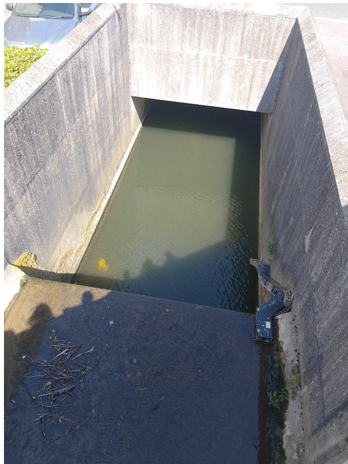
Photo 12 The large vertical drop and next culvert – right hand channel. An elver pass has been installed to the side of this.
